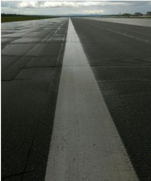
Figure 3.1. Edge Markings.
