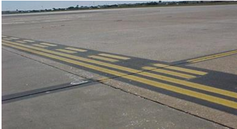
Figure 3.3. VFR Hold Position Marking.
