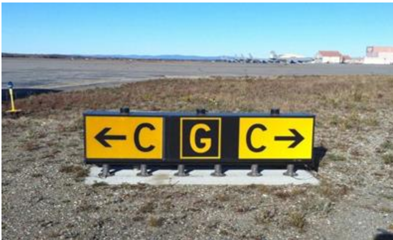
Figure 3.8. Taxiway Information Sign.
