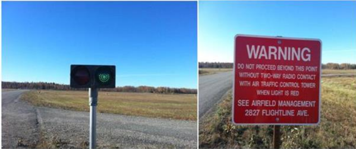
Figure 3.5. Perimeter Road Traffic Lights.
