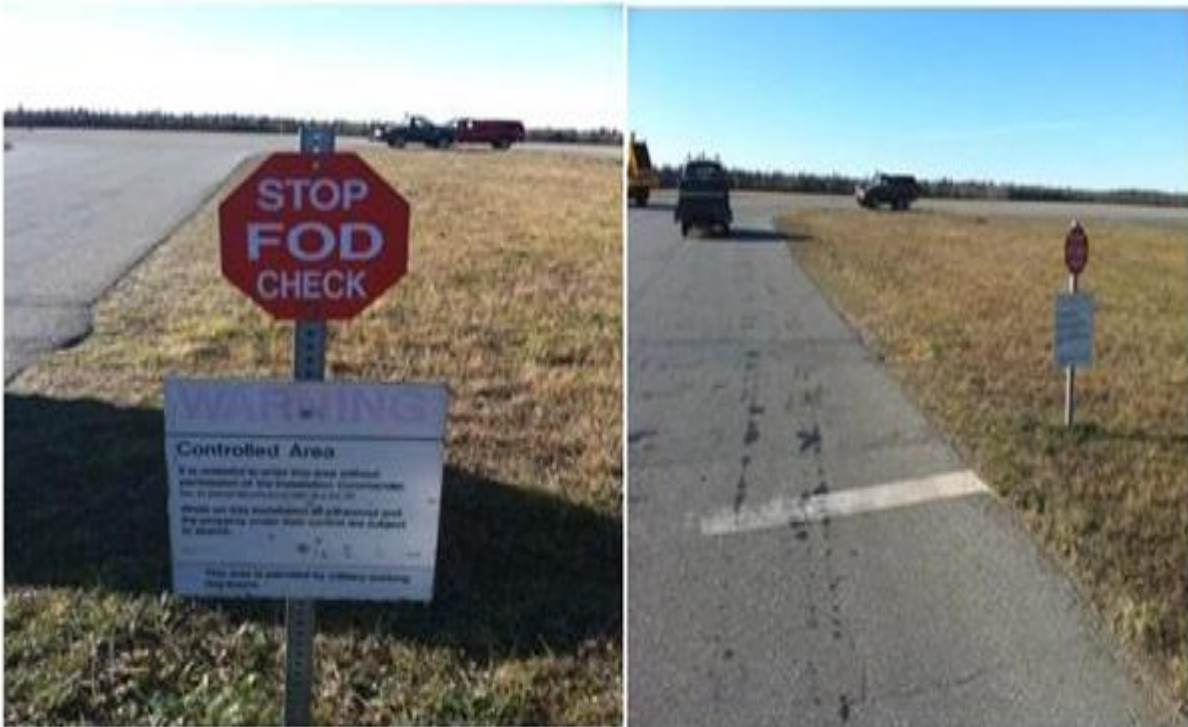
Figure 3.10. FOD Check Point Sign / Stop Bar.
