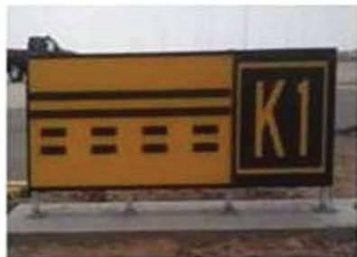
Figure A10.7. Boundary Sign for Runway Protected Area with Taxiway Location Sign
