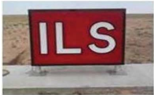
Figure A10.2. Mandatory Instrument/POFZ Hold Position Sign
