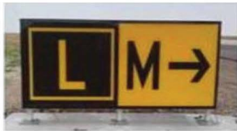
Figure A10.4. Taxiway Direction Sign with Taxiway Location Sign
