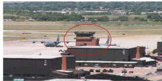
Building 122 Tower from Tower
