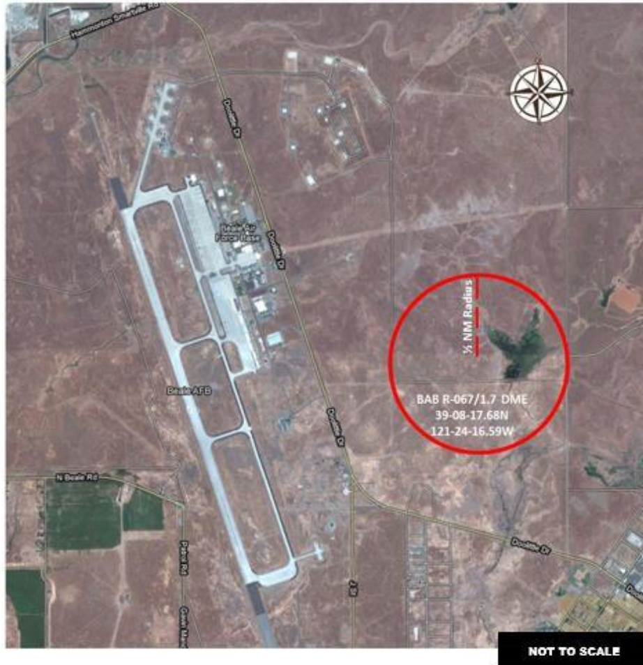
Figure A15.1. RQ-4 Termination Point.
