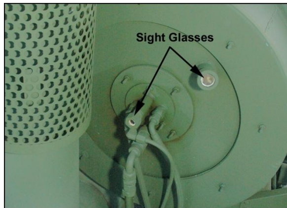
Figure 2.9. Sight Glass Assembly.
