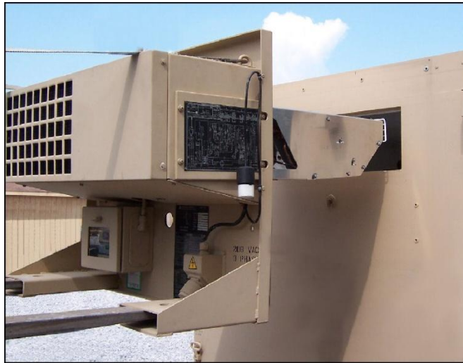
Figure 3.12. Installation of Refrigeration Unit with a Forklift.
