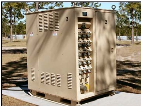
Figure 2.4. Secondary Distribution Center (SDC), Low Voltage Side.
