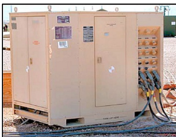
Figure 2.11. Secondary Power Cables Connected to SDC.
