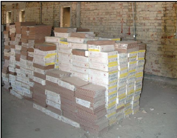
Figure 7.2. Store Weather-Sensitive Materials Under Cover
