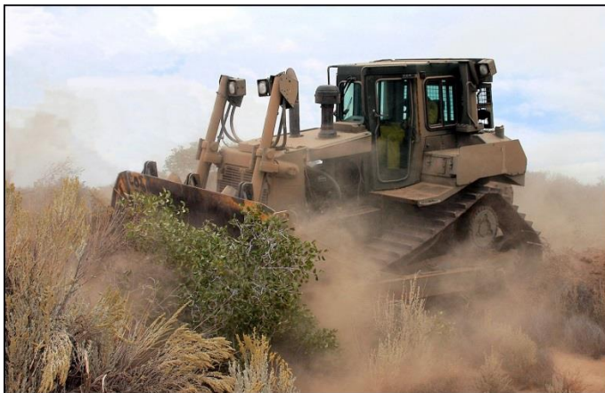
Figure 4.3. Engineers Using Heavy Equipment to Cut a Fire Break
