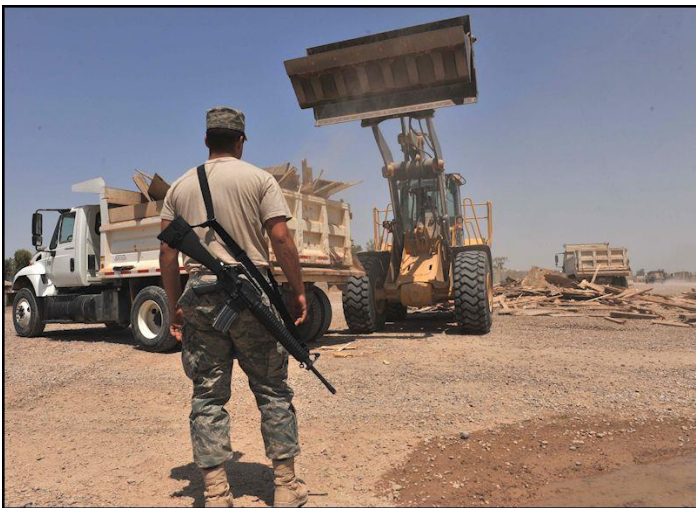
Figure 8.1. Work Party Security Help Safeguard CE Work Crews
