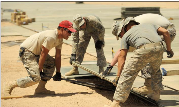
Figure 6.3 Laying AM-2 Matting at Deployed Location.
