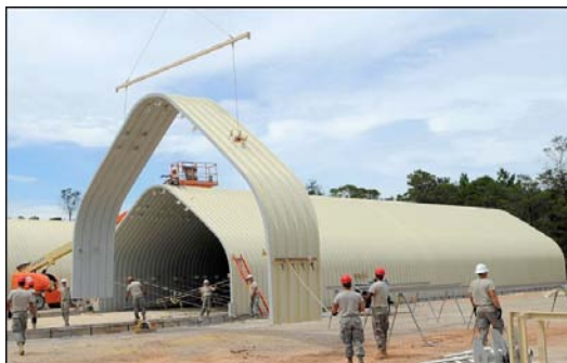
Figure 7.19. K-Span Facility Under Construction.
