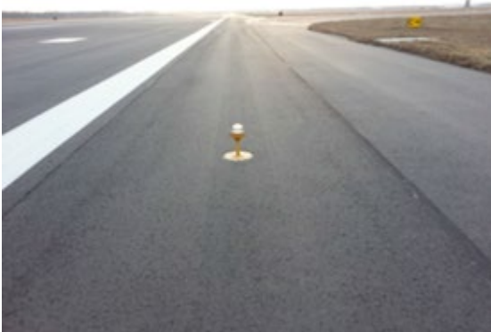
Figure 5.10. Runway Edge Lighting.
