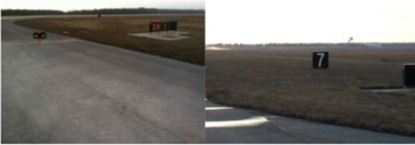
Figure 5.4. Runway VFR hold sign and DRM.
