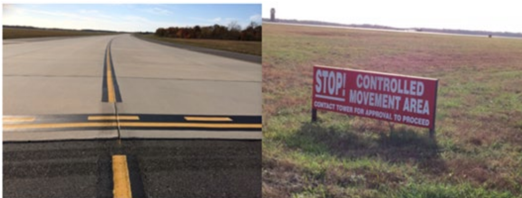
Figure 5.7. Taxiway Hotel CMA Boundary Marking and Signage.
